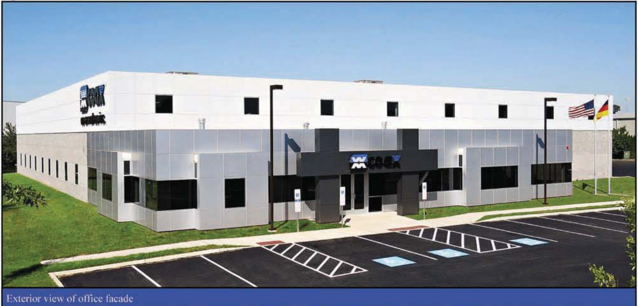
Exterior view of office facade
