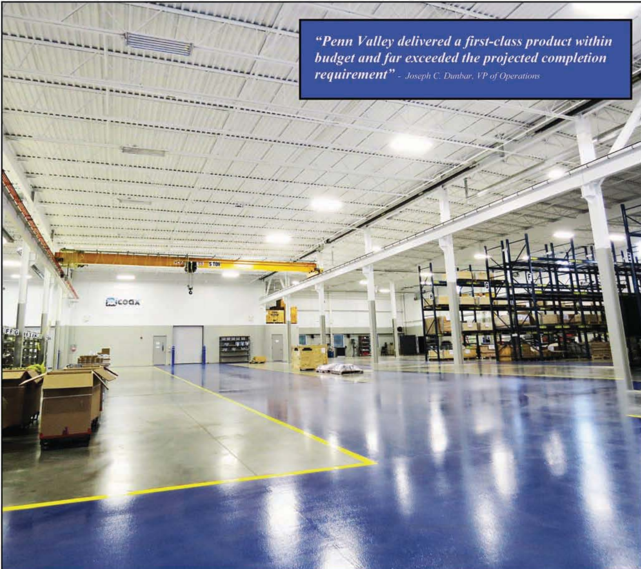
Warehouse view and crane
